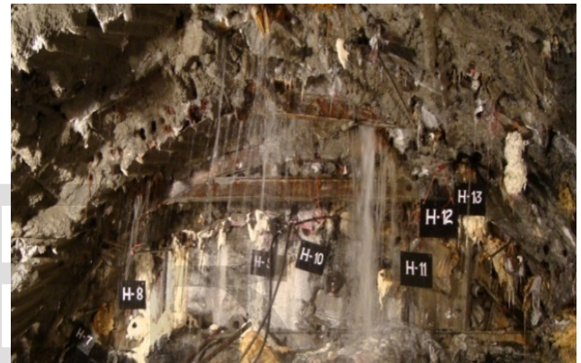
Photo: 12: PU (polyurethane) Grout, HRT Face-VI.
