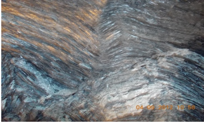
Photo: 9: The rock condition of face and the squeezing takes place the rock seems to experience high stress.
